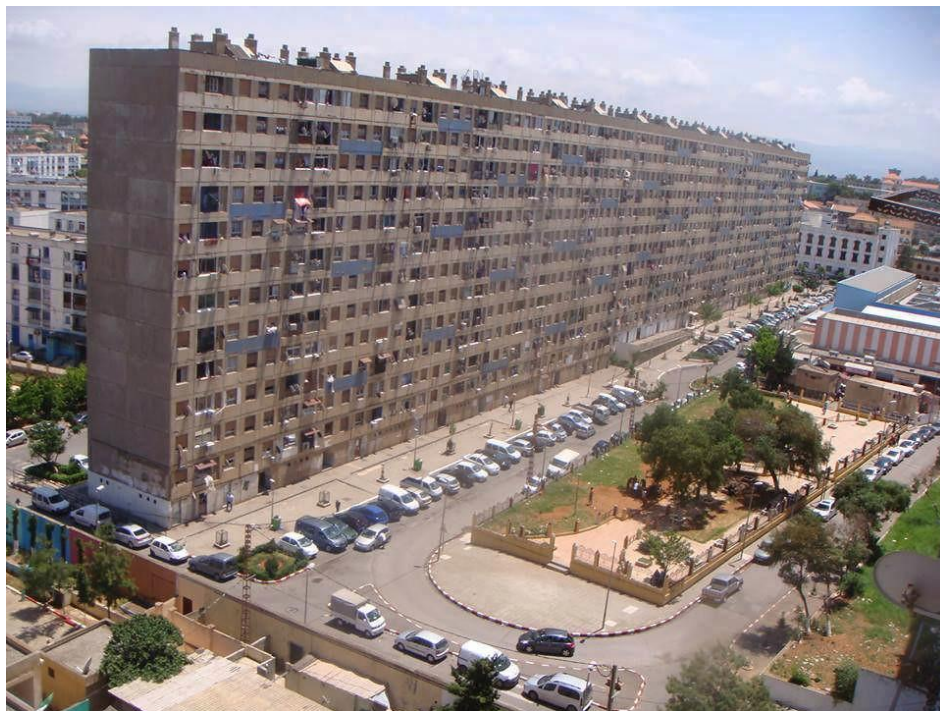
Figure 45: Rhythm, diversity, and visual aspect in the collective housing of Dunes El Harrach, Algiers
