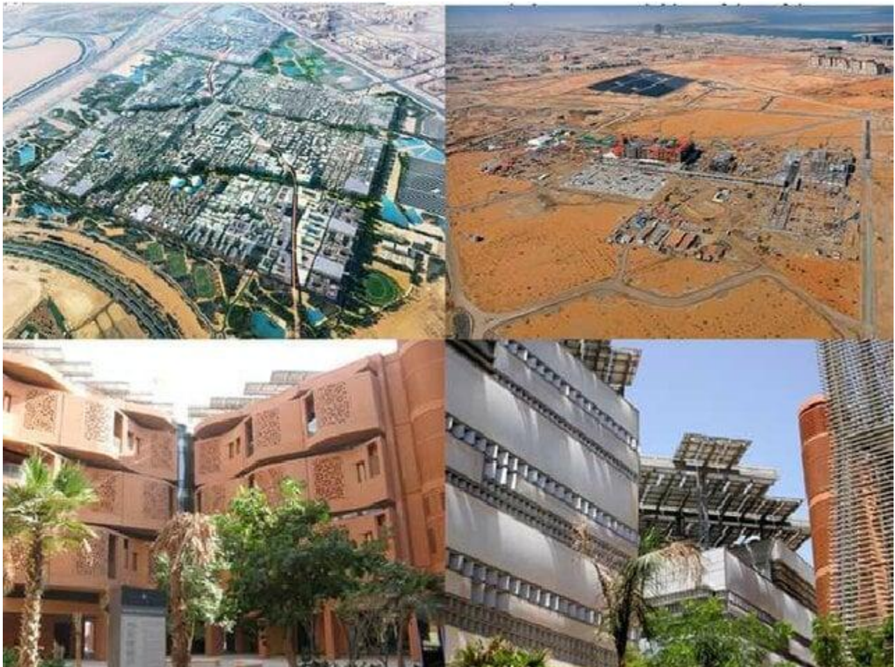
Figure 21: Masdar City as an example of how urban design responds to hot climate through shade, compact form, and water management [56]
