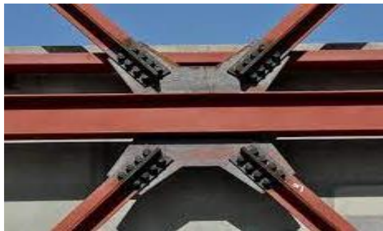
Figure IV.15: Types of bracing, stiffening of nodes [7]
