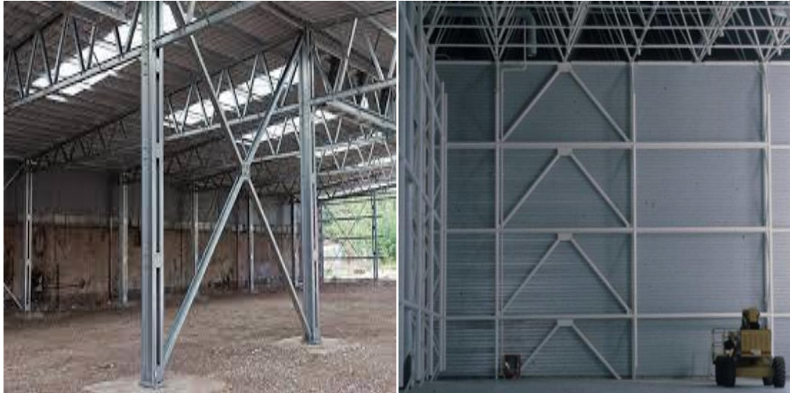
Figure IV.14: Types of triangulation bracing [5]
