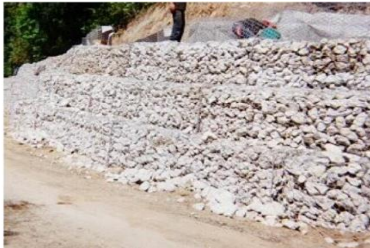
Figure 1.4 : Mur de gabion.
