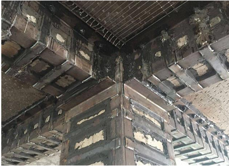
Figure II. 4 :Colle de gaine en acier.
