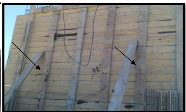
Figure.1.54. Assurer le coffrage.
