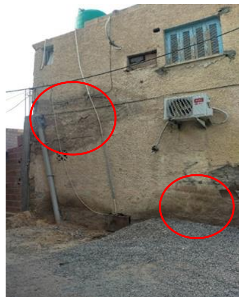
Figure 16 Clear mould spots appearing on the exterior wall of a residence in the Bab Al-Darb neighbourhood.
