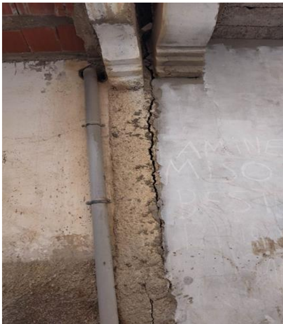
Figure2 Cracking and degradation of the exterior wall with the continuation of cracks to other parts of the house facade (Sitar Al-Muluk neighbourhood)
