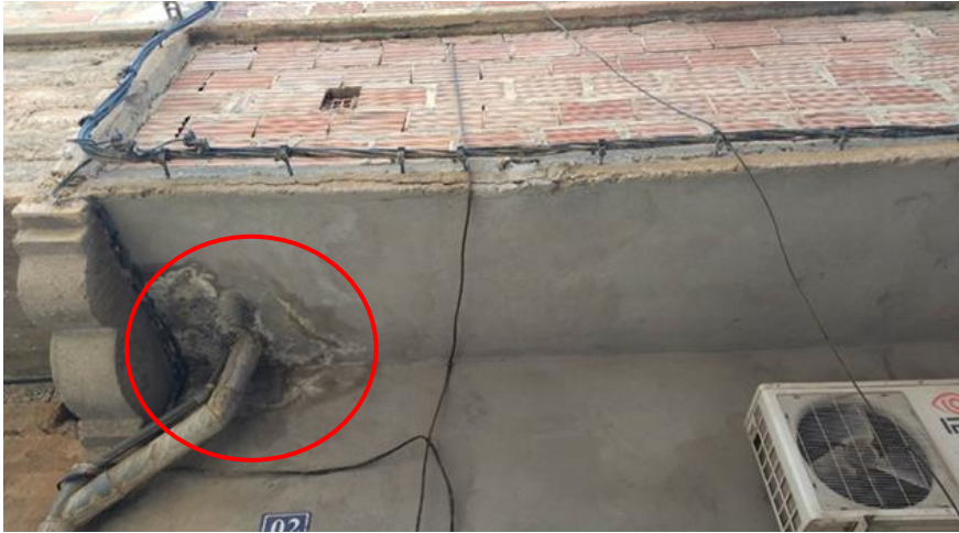
Figure9 This figure shows the leaking sewage pipe and the mould that has grown around it in the Al-Dhala neighbourhood.
