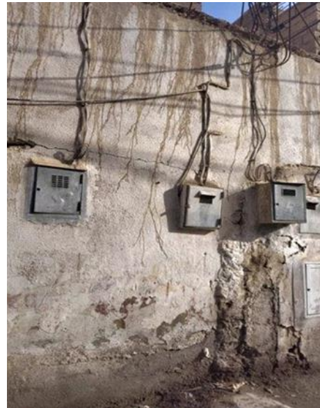
Figure 20 Shows exposed electrical and gas wires and the degradation of the housing wall in the Al-Masid neighbourhood.
