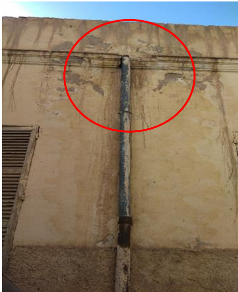
Figure8 Horizontal cracking, mould appearance, and paint deterioration (SAlmahatta neighbourhood)
