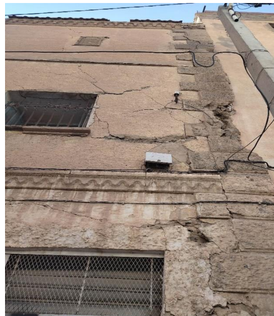
Figure3 Vertical crack at the level of the dividing column between the two residences (Bou Said neighbourhood)
