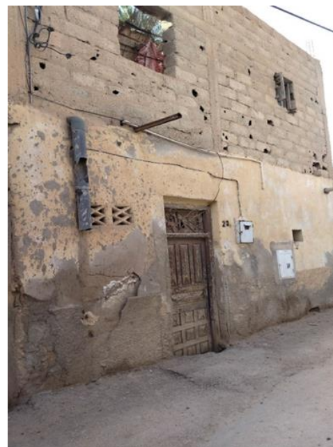
Figure 9 The degradation of the facade due to the ageing of materials in the Al-Masjid neighbourhood is evident.
