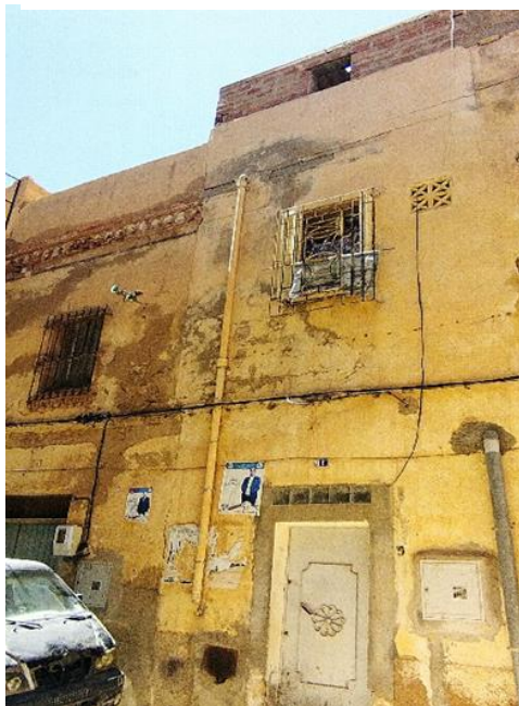
Figure 8 The paint damage due to lack of maintenance is evident in the Haret Al-Wad neighbourhood.
