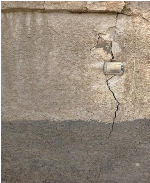
Figure12 Deformation in the installation of electrical equipment and the appearance of a horizontal crack in the external wall of the residence in the Khobzi neighbourhood.
