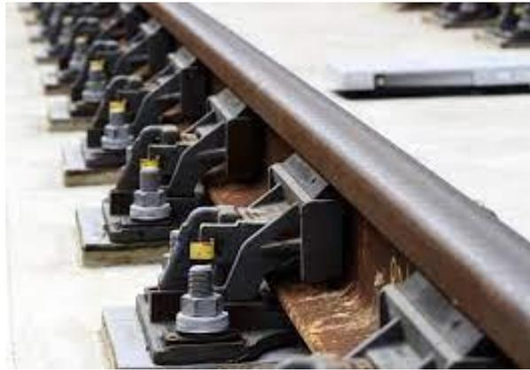
**Figure 1.15 :** Fixation des rails.
