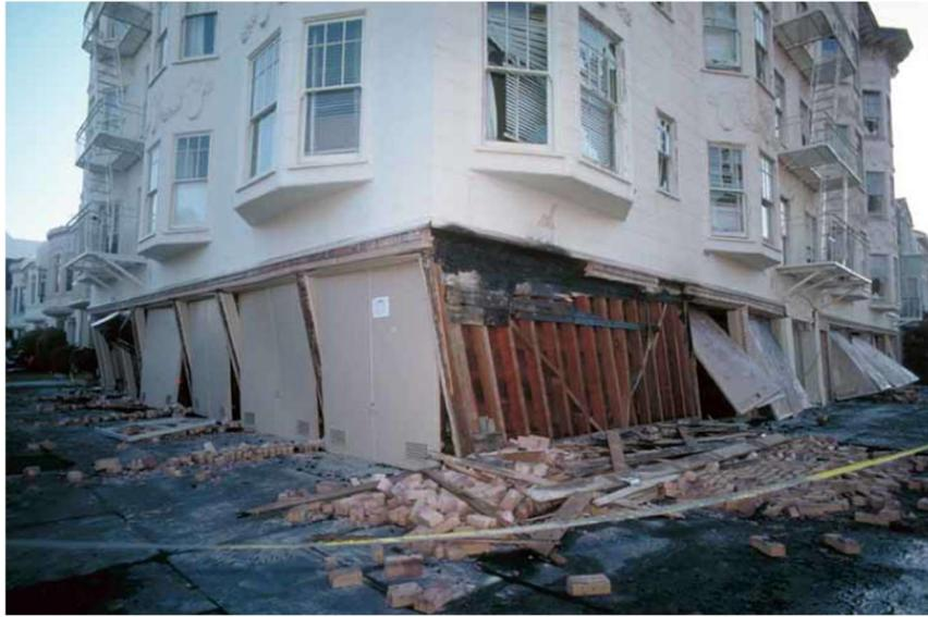
**Figure 1-5 :** The absence of sufficient shear walls at the garage level of the building resulted in total damage during the 1989 Loma Prieta earthquake
