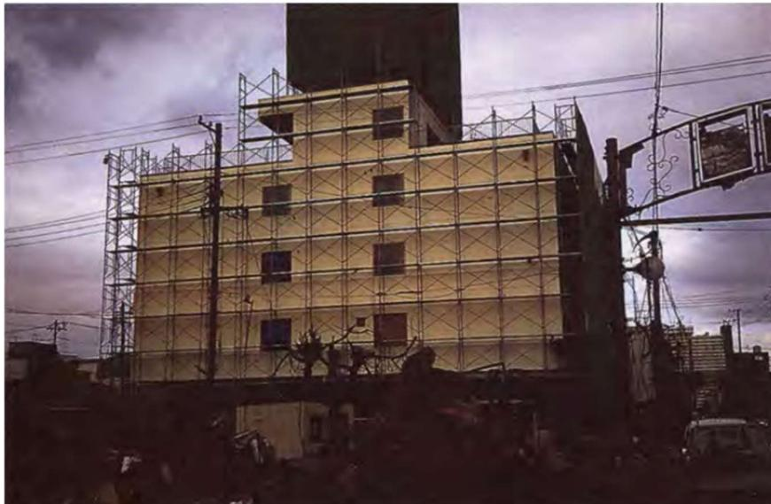
**Figure 1-4:** An undamaged hospital building made of reinforced concrete shear walls stands unaffected in the midst of extensive fire damage during the 1995 Kobe earthquake (Ghosh, 1995).
