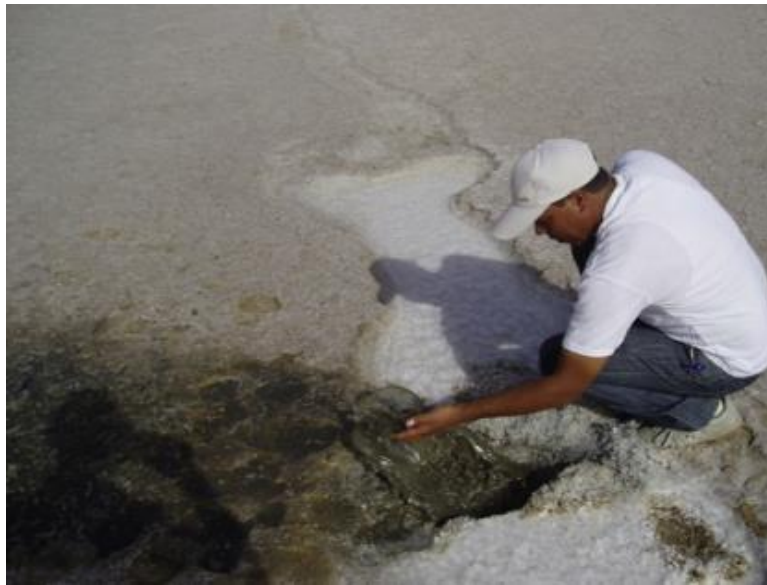
Figure 1. Example of the locally weak zone: Chott El Hodna in Algeria (Benmebarek et al. 2015),
