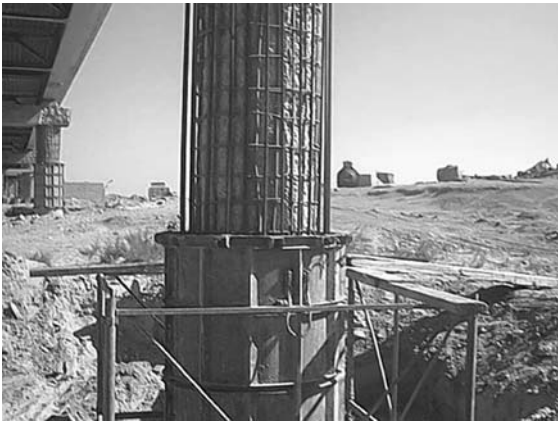
Fig. 4 Repair of pier.
