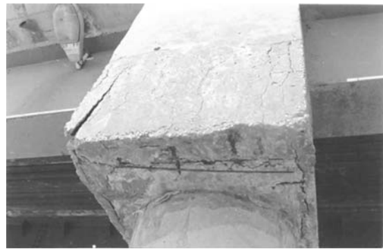
Fig. 3 Degradation of the cross beams.
