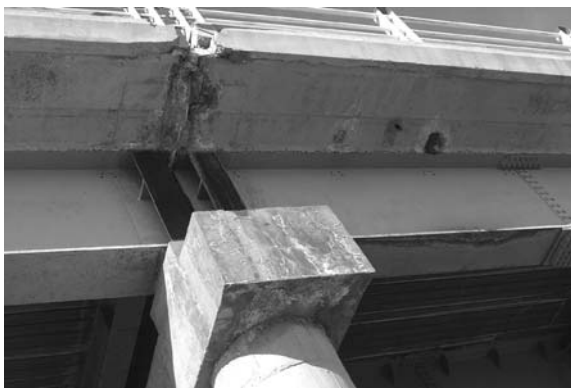
Fig. 7 Heavy water flow traces indicating very poor jointing and defective rain water.
