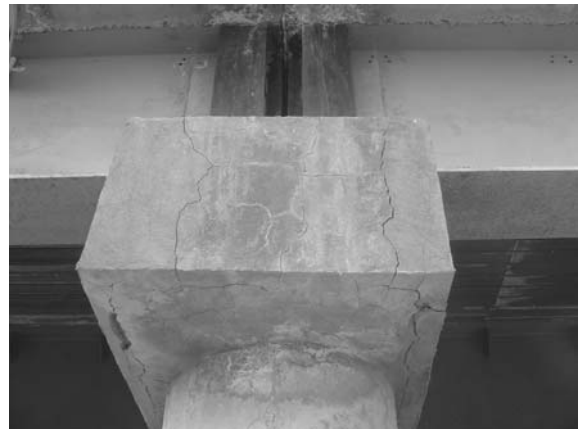
Fig. 5 Multi-directional cracking of the concrete. After repair.
