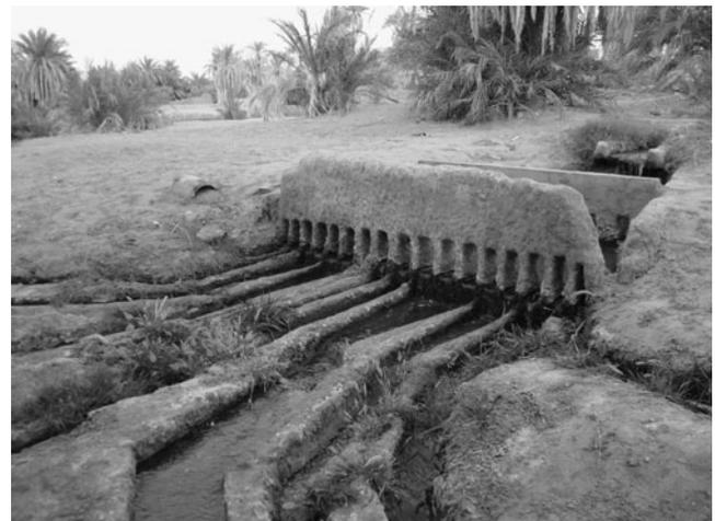
**Fig. 3** The large comb (flow splitter) of the foggara El Meghier (Timimoun) (photography Remini and Achour 2008)
