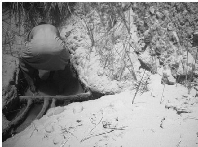
**Fig. 17** A periodic cleaning of the foggara Kasria of Badou (photography Remini and Achour 2008)
