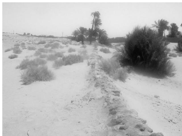
**Fig. 18** Coverage of seguia by flat slabs of rock, a way to fight against sand (photography Remini 2007)
