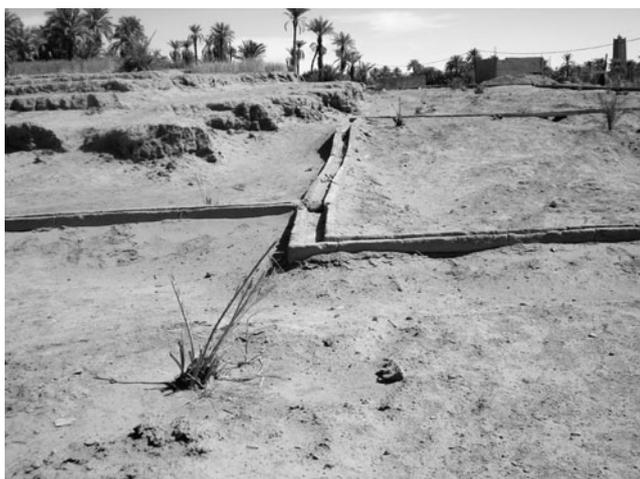
**Fig. 16** A portion of the network of the foggara seguia El Méghier abandoned (photography Remini and Achour 2008)
