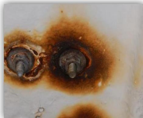
Figure (I.3): Schematic representation of crevice corrosion.
