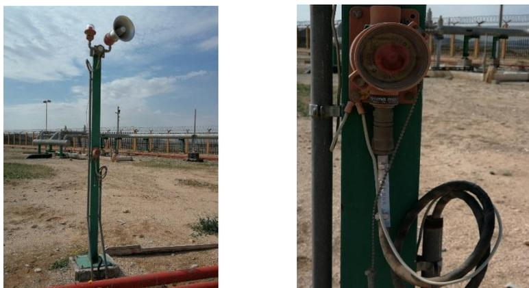
Figure III.6 : Button poussoir alarme incendie (BP-xxx) /DI.
