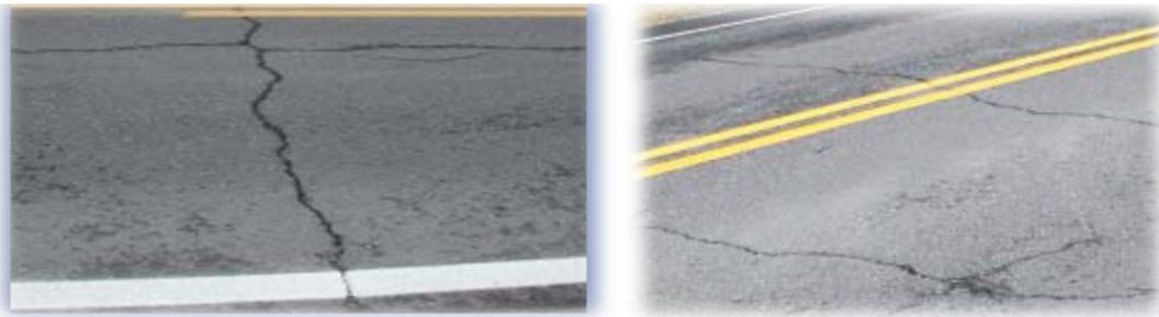
**Figure 1.2 :** Fissure transversale
