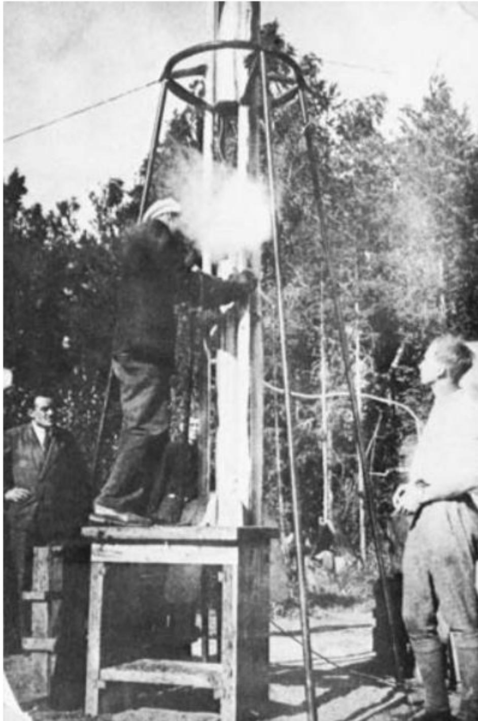
**Figure A.3.** Members of Russian amateur rocket group GIRD work on the first Soviet liquid propellant rocket (left to right): Sergei Korolev, Nikolai Yefremov and Yuriy Pobedonostsev. The rocket reached an altitude of 400 m on 17 August 1933 [NASA/Asif Siddiqi].
