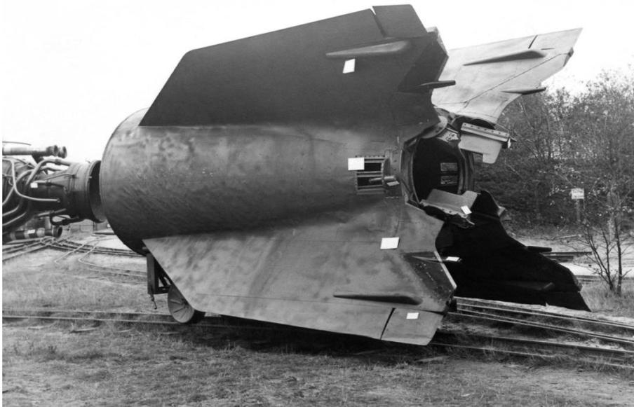
**Figure I.31.** Four fins attached to tail section, the parts are in an assembly rail.
