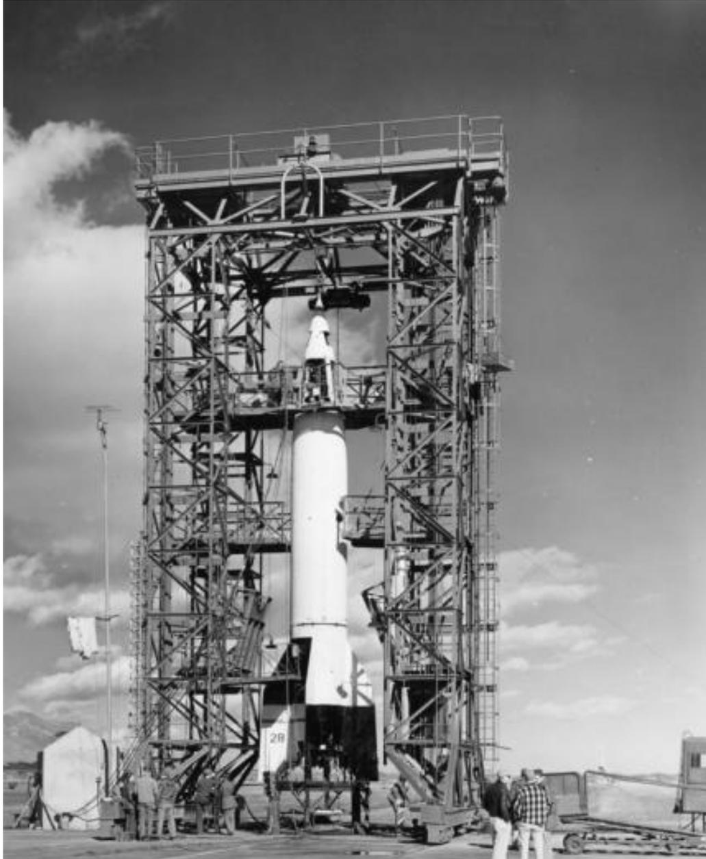
**Figure A.4.** V-2 on launch pad. The German V-2 was a key element of early U.S. and Soviet ballistic missile development. This V-2, at White Sands in New Mexico, served as a test bed for the U.S. Army and allowed engineers to experiment with several new technologies. (Courtesy, U.S. Army).
