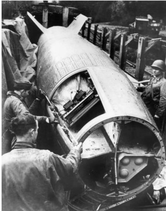
**Figure I.26.** American soldiers inspect a V-2 rocket captured intact in April 1945.
