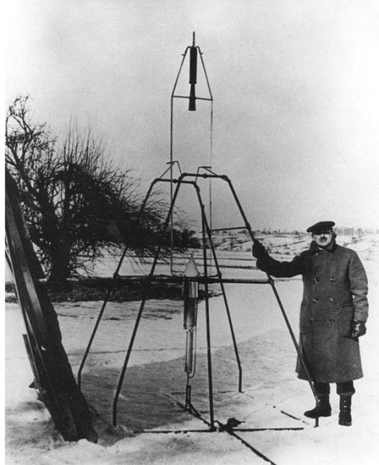
**Figure I.14.** Robert H. Goddard and a liquid oxygen-gasoline rocket at Auburn, Massachusetts [NASA].
